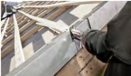
Carbide technology enables you to effortlessly cut through mounted profiles in outdoor areas.
